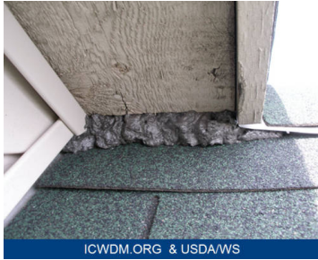
Bat entry in roof sealed with Todal foam
